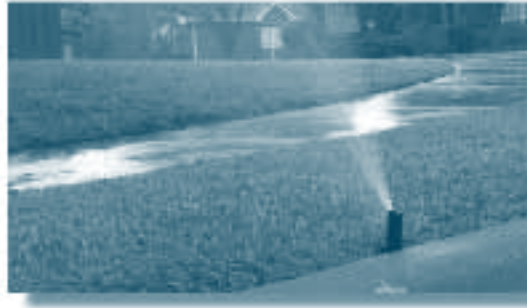
Conserve Water optimize water schedules and durations
